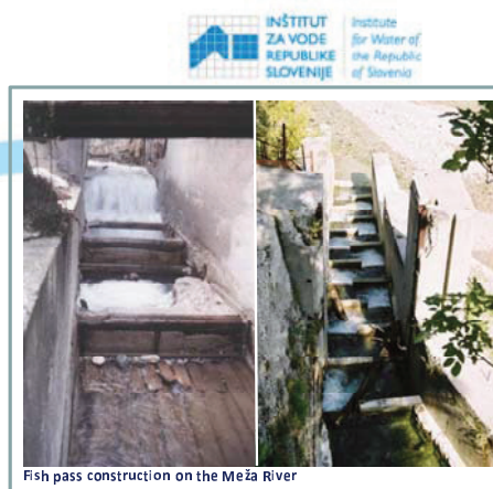
Fish pass construction on the Meža River
