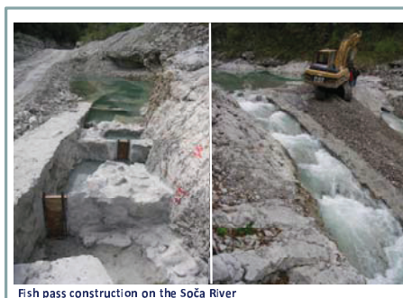
Fish pass construction on the Soča River
