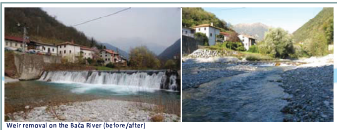
Weir removal on the Bača River (before/after)
